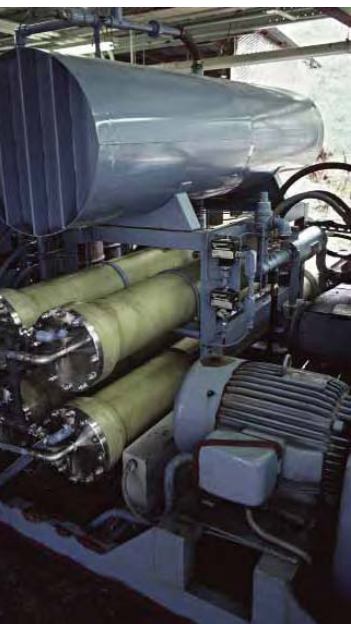
Reverse osmosis desalination unit in the Virgin Islands, United States
