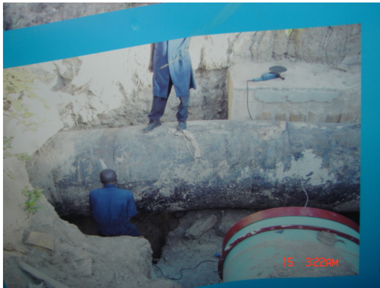
Figure 2: Technicians repairing/replacing burst pipe
