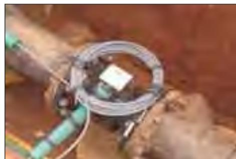
**Picture 5.2** Electromagnetic flow meter installed in Bangalore
