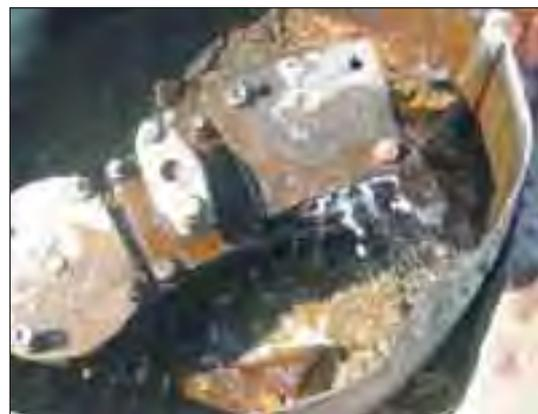
**Picture 5.7** Valve leaking near Bhongadwar
