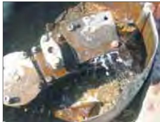
**Picture 5.7** Valve leaking near Bhongadwar
