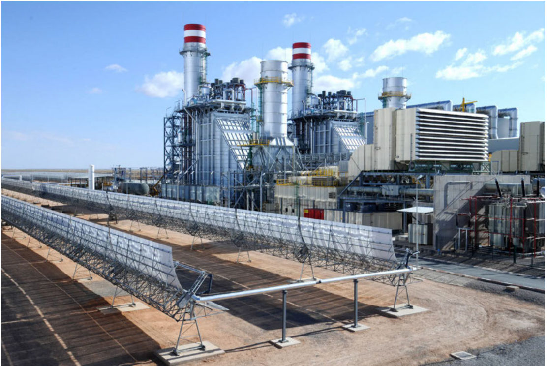
Ain Beni Mathar Integrated Combined Cycle Thermo-Solar Power Plant, Morocco. © World Bank/Dana Smillie
