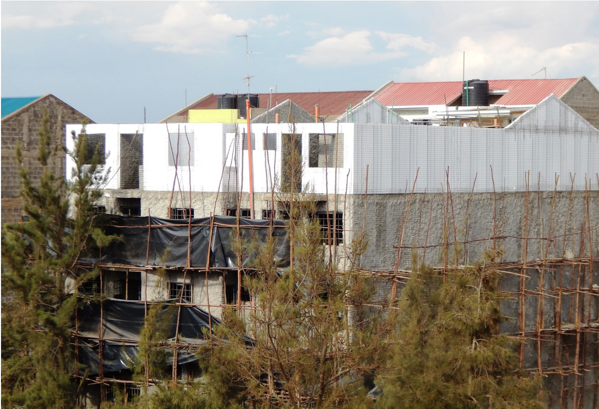
Housing construction using alternative building technologies, Nairobi. © Baraka Mwau/UN-Habitat
