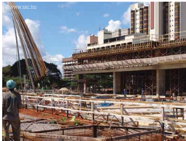
Urban construction site
