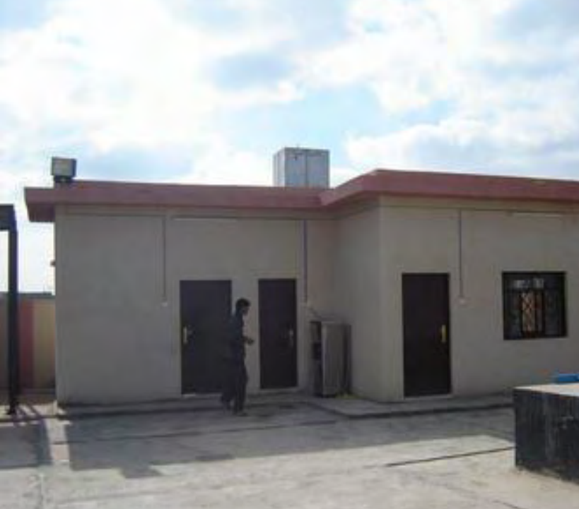
Pumping Station in / Samawa
