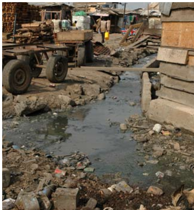
Sewerage Problem in the informal settlements in Old Fadama, Accra, Ghana. © Suzi Mutter, 2005.
