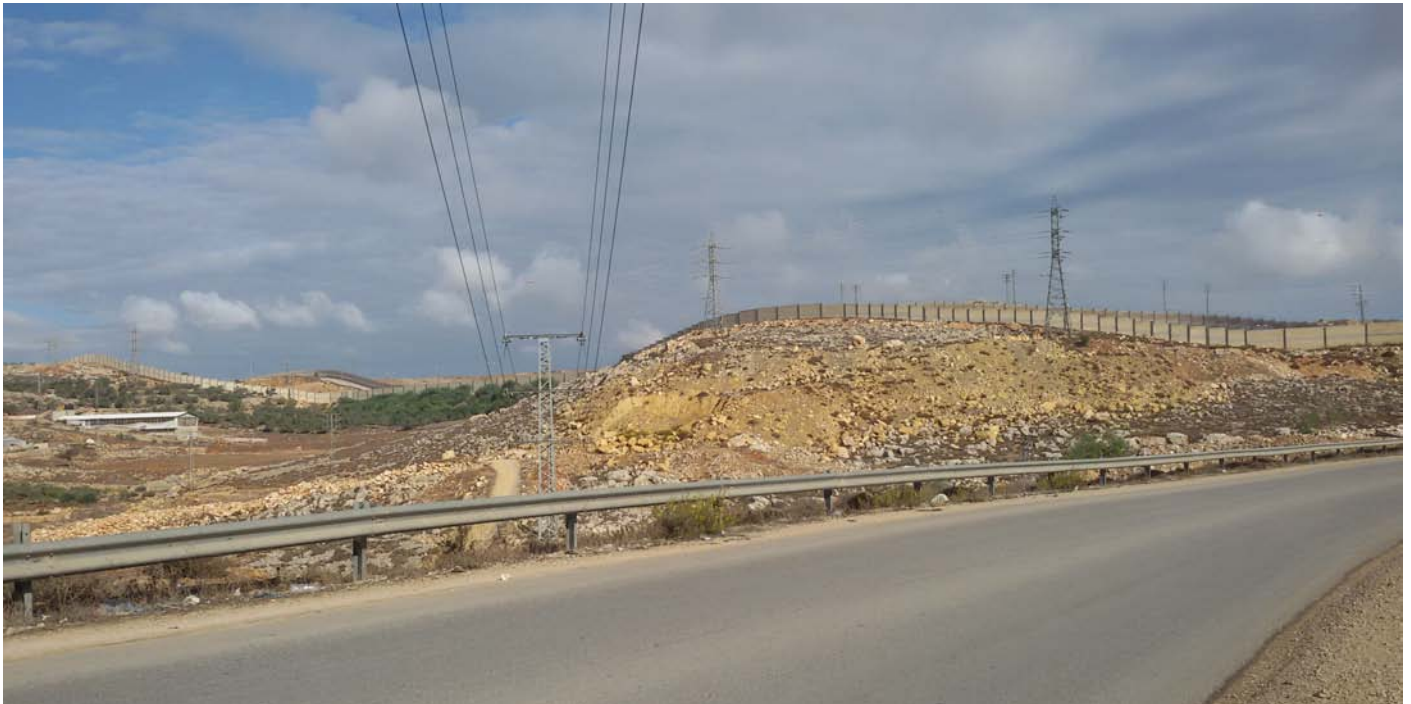
Flanking walls and restrictive access to the Israeli Highways are serious mobility barriers and development impediments for Palestinian communities
