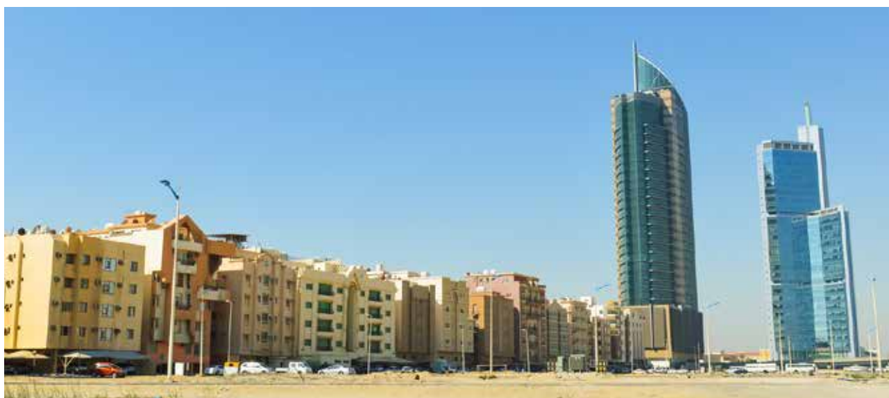
New construction on Prince Salman Road © Flickr/Francisco Anzola
