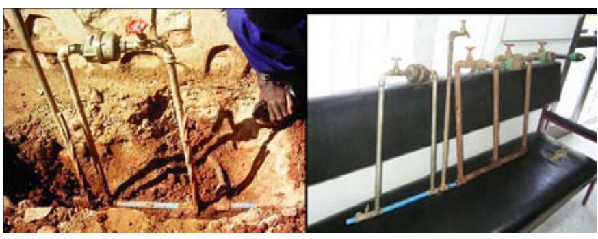
Plate 1: Pictures of a meter by passing in the field
