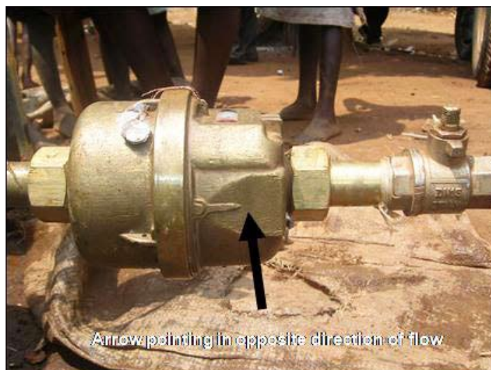
Plate 5: Example of a meter that has been reversed
