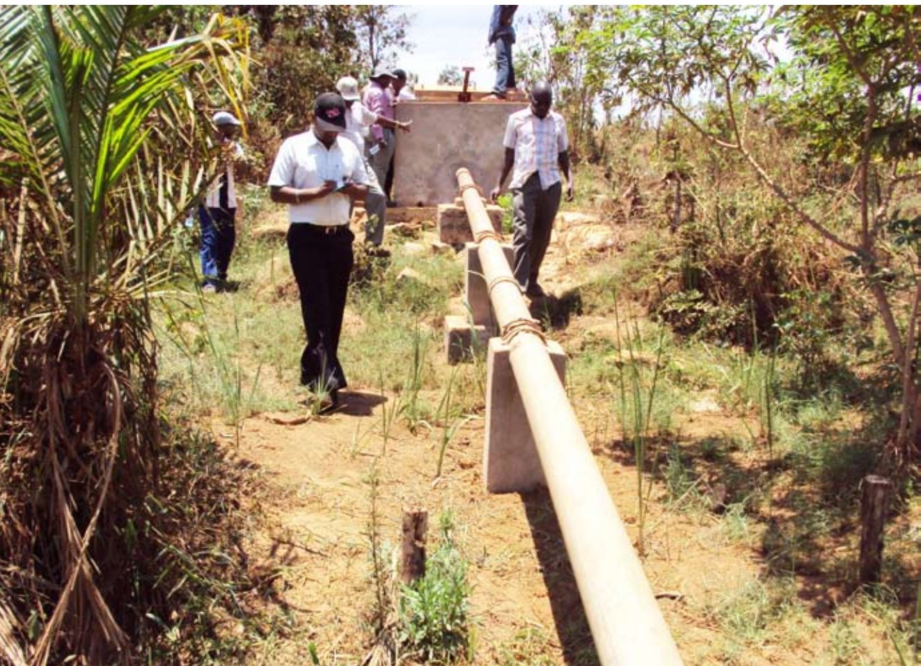
Water pipes maintenance and illegal water reduction exercise. Photo © UN-Habitat
