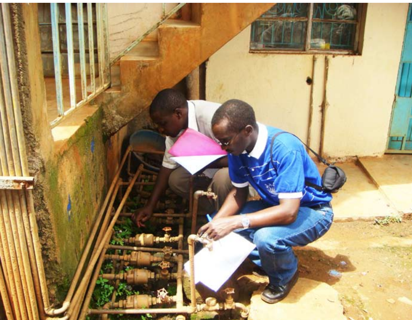
Investigation of house water connections. Photo © UN-Habitat
