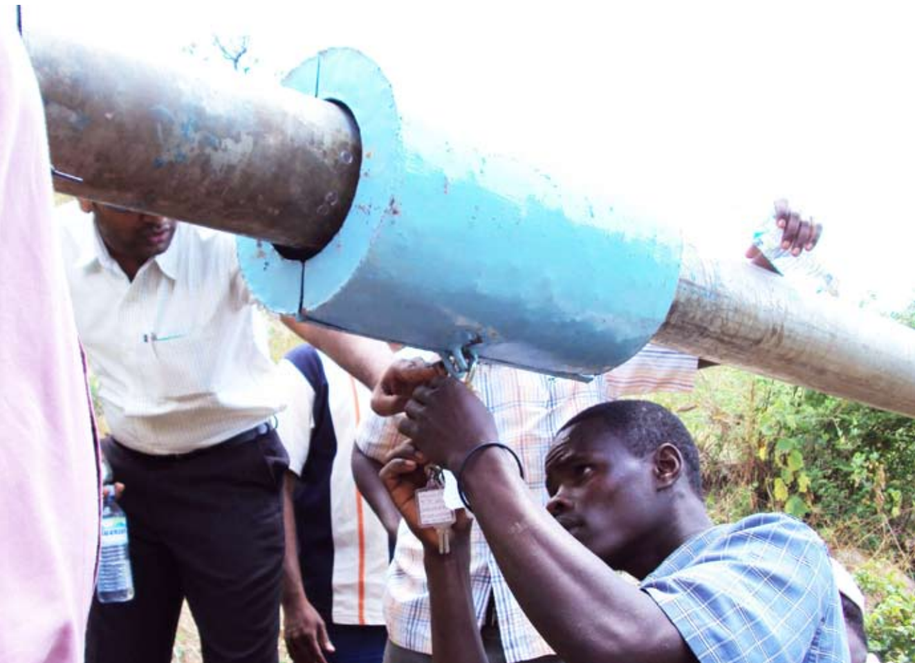
Water pipe maintenance. Photo © UN-Habitat
