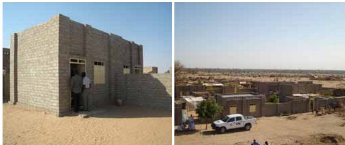
Figure 14. Construction of Pilot Demonstration Buildings in Darfur
