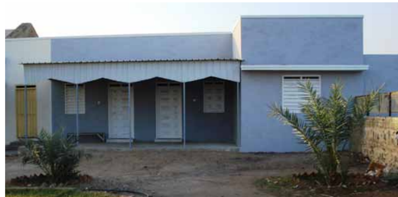
Figure 15. Construction of new offices for the teachers in the eastern region
