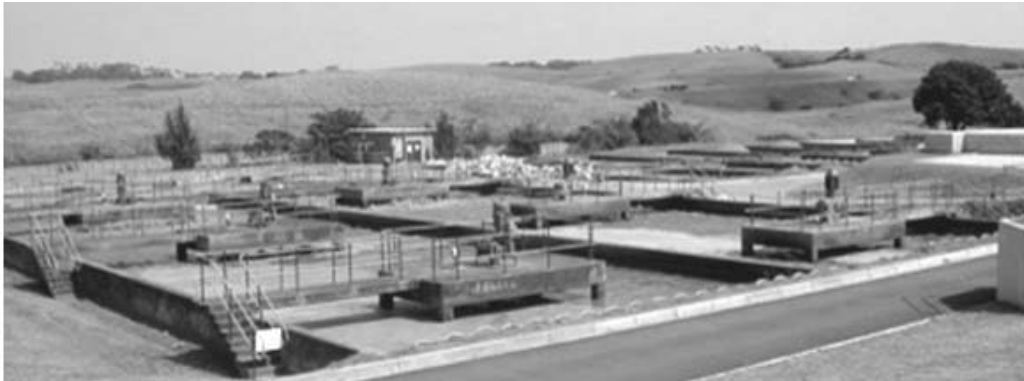
FIGURE 8: Ilembe District Community Water and Wastewater Plant
