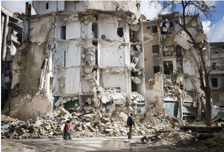
Bombed out building in Aleppo, Syria. Photo© UN-Habitat
