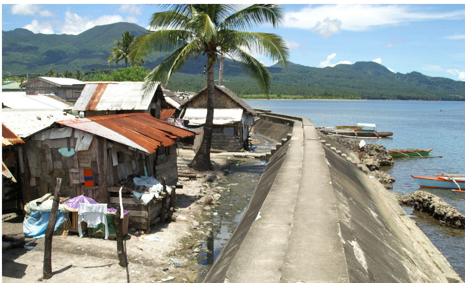
Protective seawall in Sorsogon, Philippines ©UN-Habitat/Bernhard Barth
