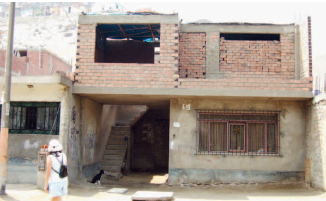
Rental units under construction in informal settlements in the periphery of Lima, Peru.
