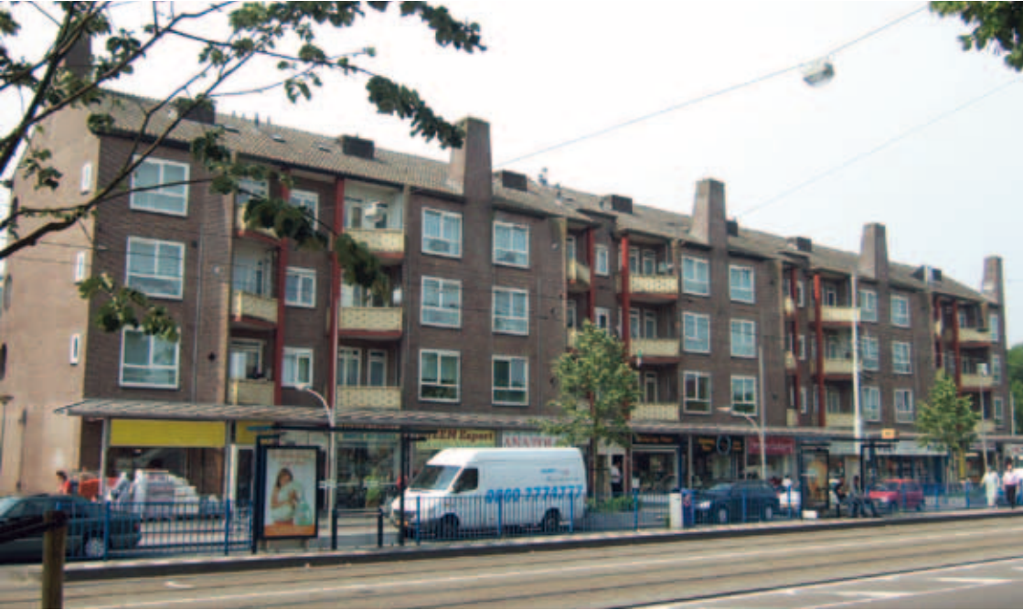
Social Rental Housing produced and managed by Dutch Housing Association, Amsterdam, The Netherlands.
