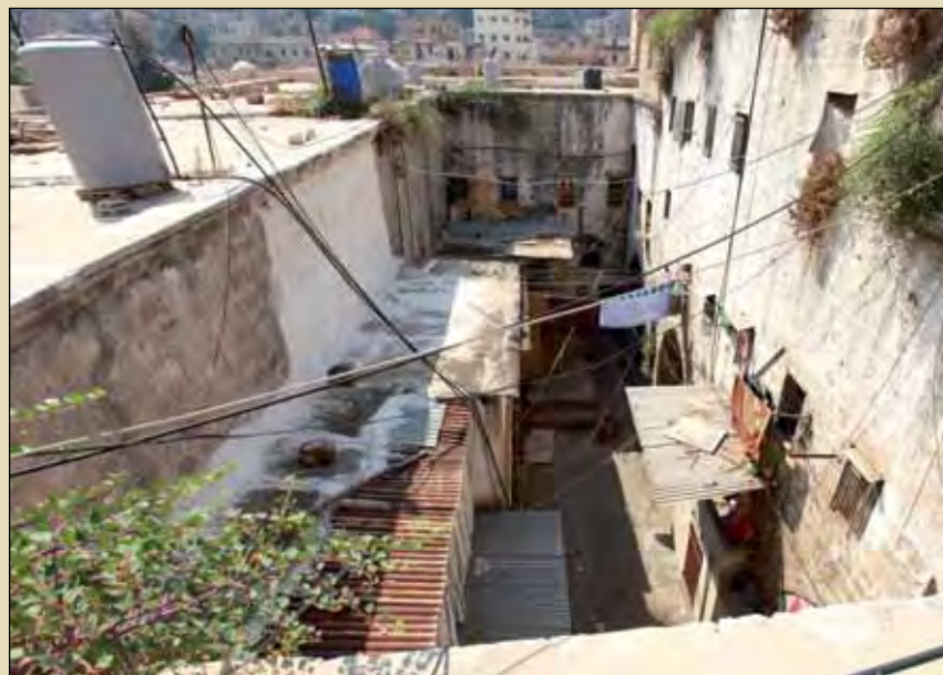
Ad-hoc electricity connections in the old quarters of Tripoli city.
