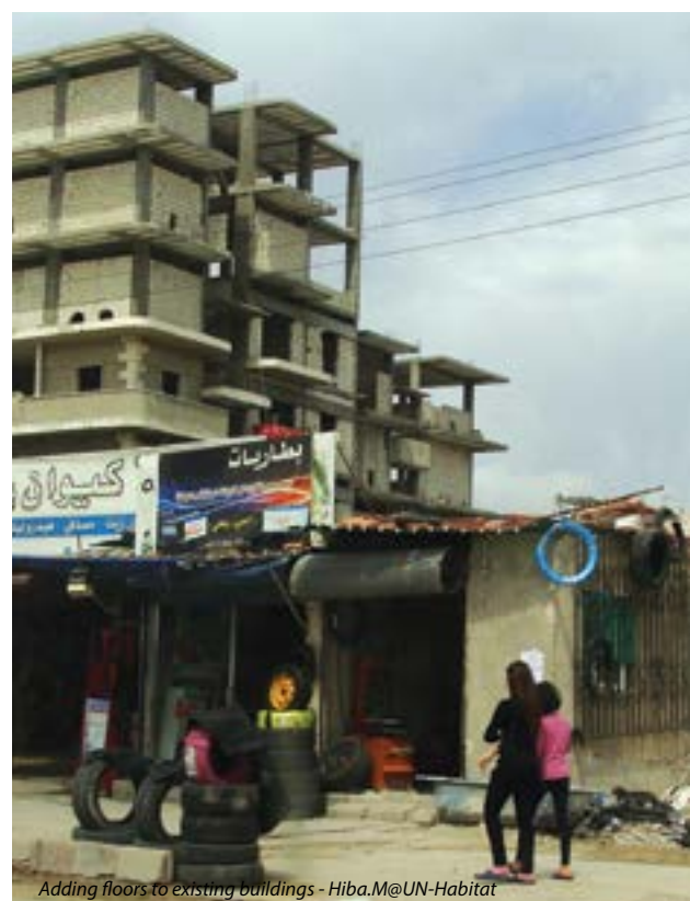
Adding floors to existing buildings - Hiba.M@UN-Habitat
