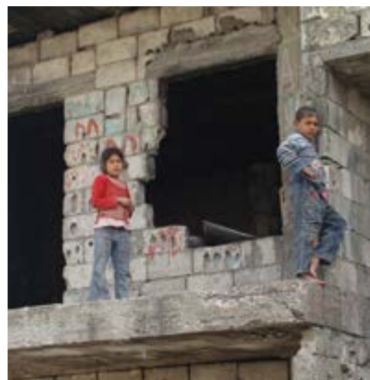
A family living in an unfinished building at Al Quds neighbourhood. Hiba.M@UN-Habitat 2014
