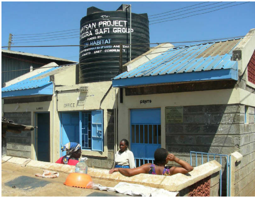
Photo 11: New sanitation blocks not only provide good quality basic water and sanitation services, but also provide a structure for community organization and for revenue generation. Funds generated by the sanitation blocks are controlled by the group members and may be used for mortgage savings.
