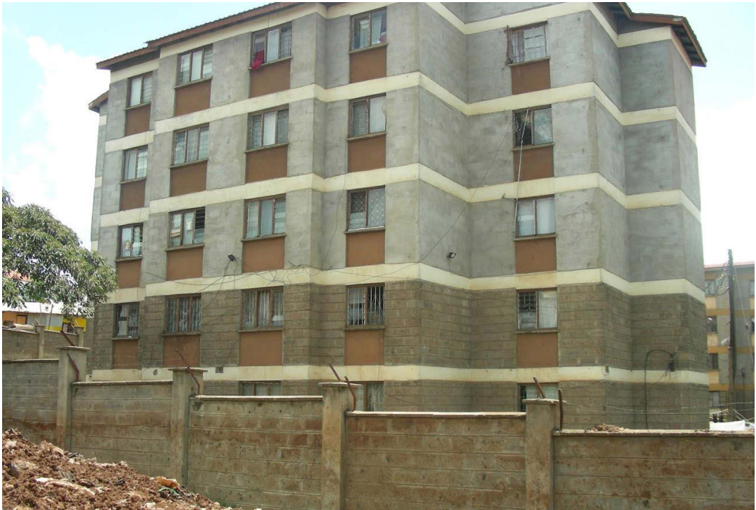
Photo 15: The Nyayo Highrise Project: adjacent high-rises that involved displacing Kibera residents, but did not lead to providing new housing for them (hence, the legacy of suspicion).
