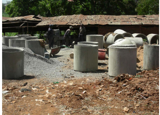
Photo 10: Making materials for the project on site employs and trains locals but may slow progress and possibly make quality control more difficult.
