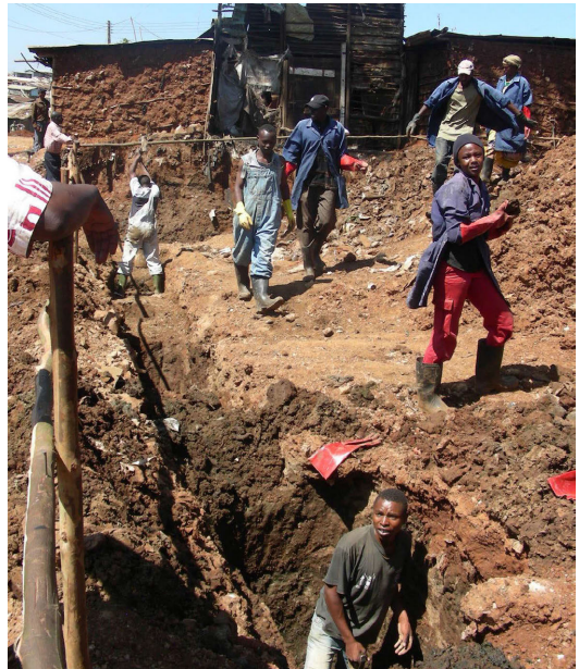
Photo 7: Manual work employs people from the community but is slower and more difficult to plan and manage than a job done by a mechanical digger.
