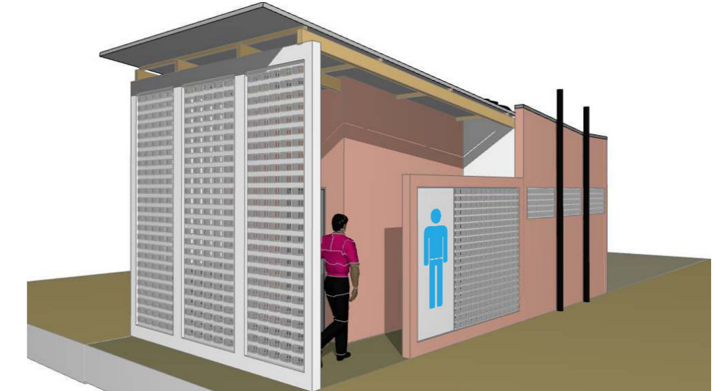
Left: An example of building with sand-filled plastic bottles. Above: Design concept for the Sinay public toilets.
