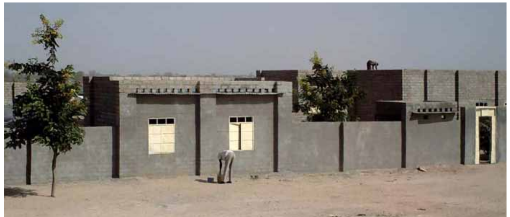
RIGHT: UN-Habitat / UNHCR - Slum Upgrading and Sustainable Housing Development - Sakali / South Darfur. © UN-Habitat
