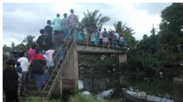
Pedestrian bridge access to Vatuwaqa settlement
