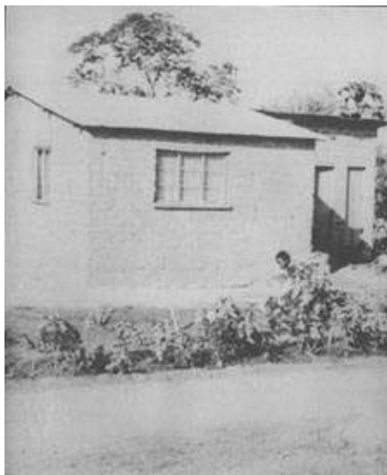
Figure 3.4. Low-cost houses using stabilized-soil walls. The blocks were made by the families who built the houses and were stabilized with 4 per cent cement. Even though left unrendered there was no sign of deterioration after eight years (Kafue, Zambia).
