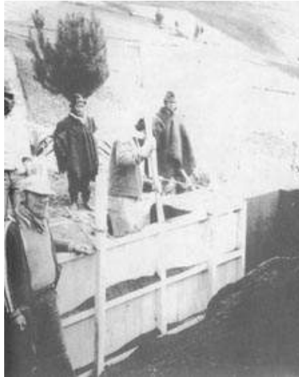
Figure 3.1. Rammed earth is a walling technique still widely used in the Andes and elsewhere. It provides excellent insulation with very little embodiment of purchased energy.
