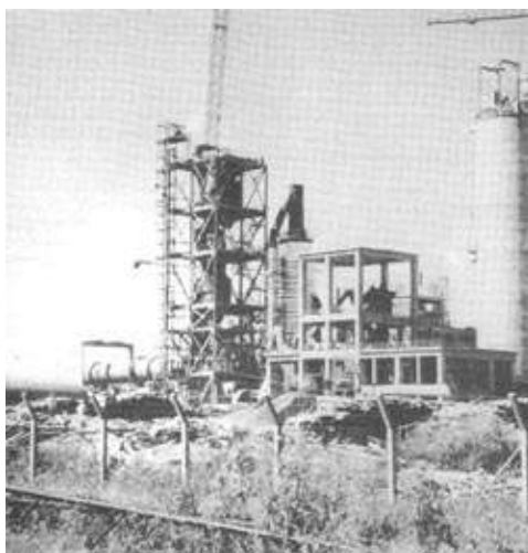
Figure 2.3. Cement kiln under construction. Large-scale cement plants typically have an economic minimum output of 2000 tons per day. In a country with a low consumption of cement, large amounts of energy are used both in production and transport (Mbeya, United Republic of Tanzania).
