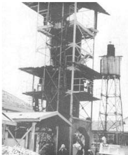
Figure 2.4. Lime can be economically manufactured at a much smaller scale than cement, appropriate to the needs of a predominantly rural population. Shaft kilns can have a high energy efficiency (lime kiln in Indonesia).
