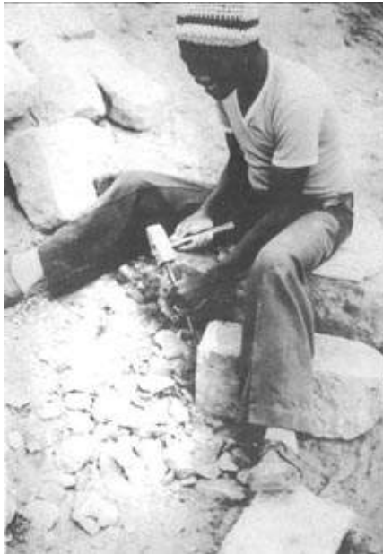
Figure 2.10. Where it is available, stone is a very low-energy building material, which often needs only quarrying and shaping, as here near Nairobi in Kenya.
