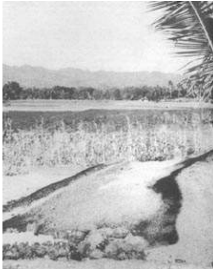
Figure 2.16. Rice-husk ash can be used as a pozzolanic additive to mortars and plasters, reducing the need for cement, and lowering the embodied energy requirement (Yogyakarta, Indonesia).
