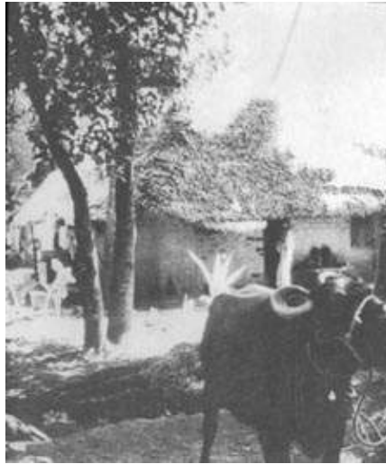
Figure 3.9. Houses with thatched roofs and earthwalls have a very low energy content, but require frequent maintenance. Replacing such houses by houses built of materials with better durability has the effect of greatly increasing the embodied energy used (Kerala, India).
