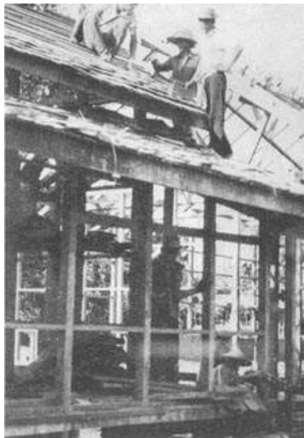
Figure 3.2. Where timber-frame housing is traditionally used, it has a very much lower energy requirement than walling using brick or concrete-block masonry (Viet Nam).
