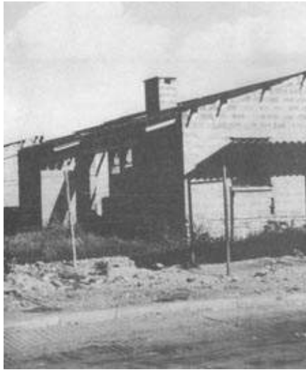
Figure 3.3. Housing built using cement-plastered concrete-block masonry with sheet roofs supported on steel roof joists is exceptionally energy-intensive compared with alternatives of comparable standard, but is still often used in public housing projects (Nairobi, Kenya).
