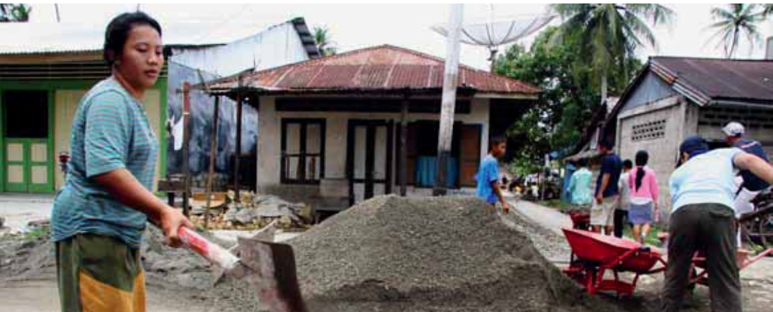
Collective self-help housing construction © UN-HABITAT
