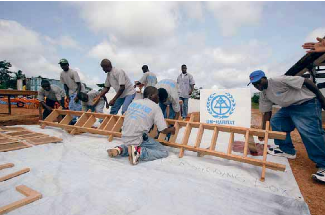
UN-HABITAT sponsored shelter construction in Liberia © UN-HABITAT
