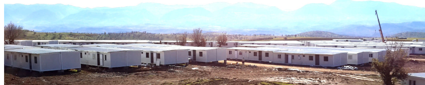
View of Dawodye project site as of 25 November 2014
