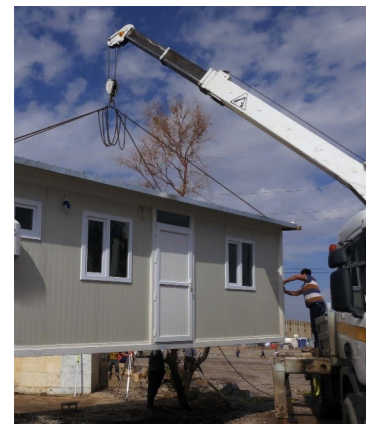
Positioning of a prefab unit in Bahrka, Erbil
