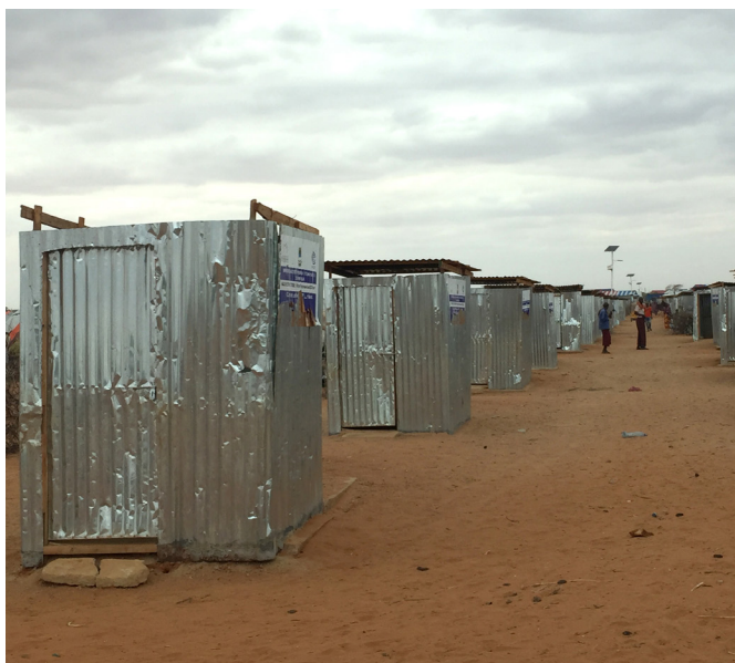
Sanitary corridor in one of the new sectors of Kabasa
