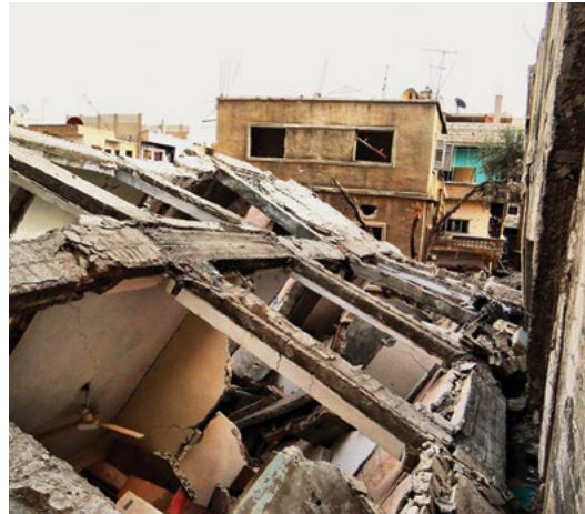
Photo 4: Damaged housing property in Al Sadd neighbourhood (2013)
