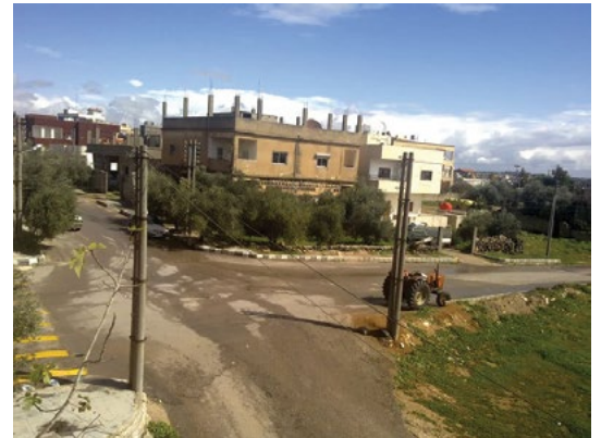
Photo 3: Dara'a Al Balad (Al Manshiah neighbourhood), the rural nature of the building typology is dominant in most of the southern city neighbourhoods.
