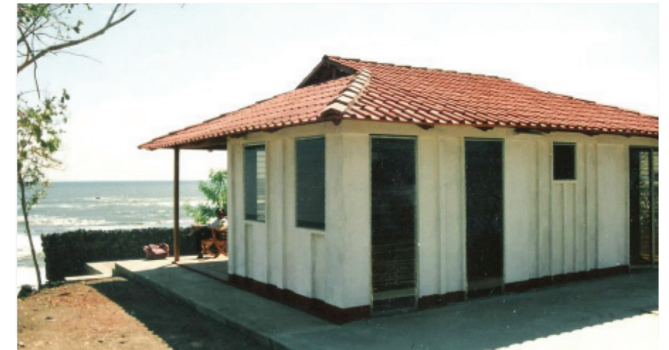
Micro-concrete roof tiles in Nicaragua. © EcoSur
