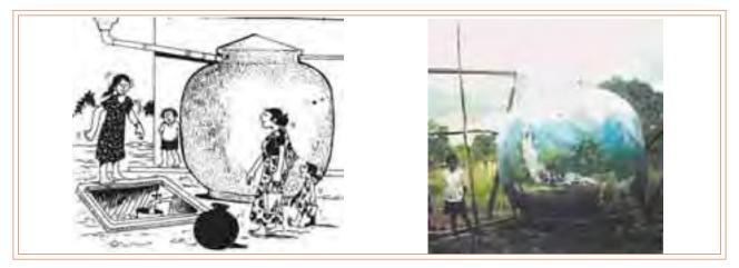
The town of Badulla is located in a hilly area of Sri Lanka. Climate: Tropical, Bimodal; Ground water sources are few and tend to be at the bottom of the hills. To reduce the burden of carrying water the local authority provided 5,000 litre ferrocement tanks, at a cost of about \$150 which are used for most household water supplies. The tanks are now being adopted nationwide for use in areas where access to other protected water sources is difficult.
