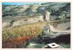
The rainwater's collected from asphaltpaved highway and conveyed to underground watercellars through a concrete lined dich
