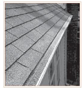
O ne example of a flat scheen over the gutter to keep large debris out of the tank. A problem with gutter scheens is that they require a btofm antenance to keep leaves and debris from piling up and blocking the scheens. Also, dirt on the leaves can still be washed into the storage tank.
