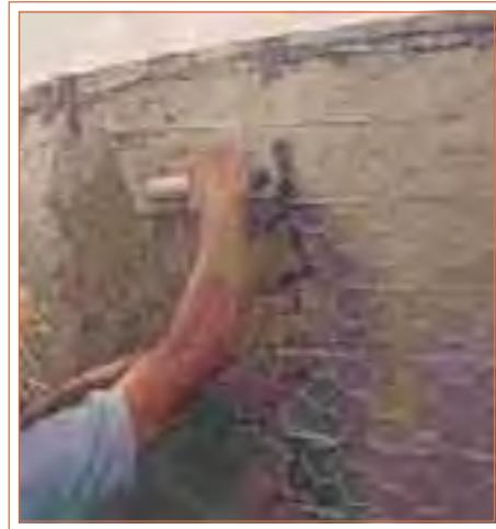
Steel sheet form wrapped by wire mesh and galvanized wire / application of first layer of mortar on top of wire
