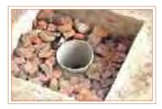
Percolation pits are made to make the rainwater directly enter into the aquifer. The structure is covered with perforated concrete slabs in paved
