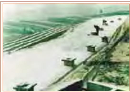
A group of water cellars and the rainwater collection field lined with concrete
