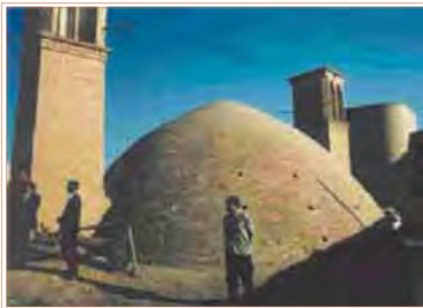
The Abanbar, traditional system in Iran (Gnädinger) as part of a traditional rainwater catchment system for the community.
