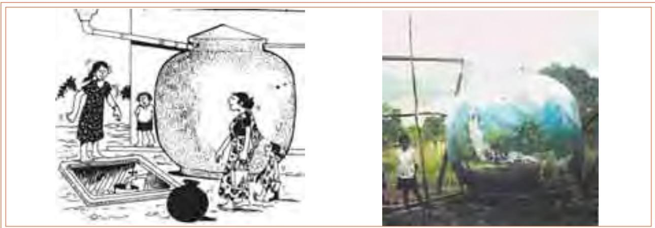
The town of Badulla is located in a hilly area of Sri Lanka. Climate: Tropical, Bimodal; Ground water sources are few and tend to be at the bottom of the hills. To reduce the burden of carrying water the local authority provided 5,000 litre ferrocement tanks, at a cost of about \$150 which are used for most household water supplies. The tanks are now being adopted nationwide for use in areas where access to other protected water sources is difficult.
