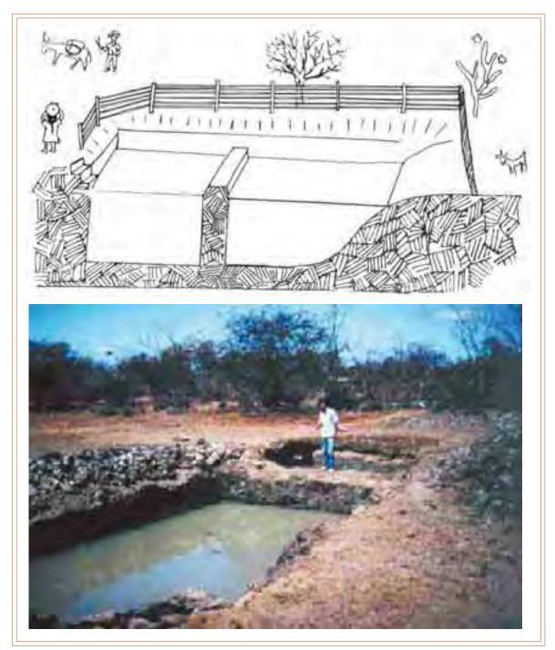
Hand dug nock cistem: In different parts of the sem iarid region there is a revival of hand-dug nock cisterns; a traditional way to harvest water for the dry season. The water is norm ally used for an in als, but after filtering can be used for drinking purposes as well
