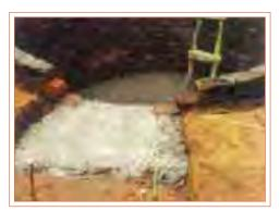
Concrete base for the inlet construction
