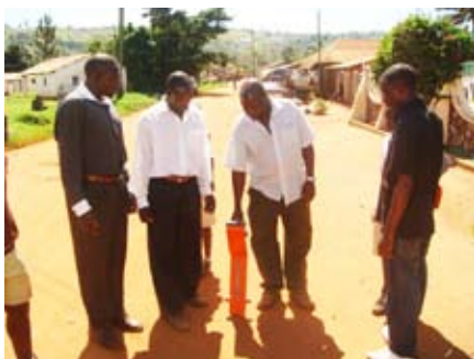
Tracing an underground metallic pipe using an electronic pipe detector
