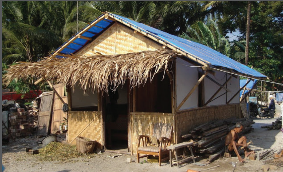
A bamboo transitional shelter built with CHF International after the 2006 Yogyakarta earthquake in Indonesia © HumanitarianBamboo
