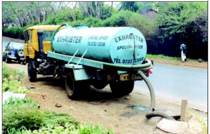
Plate 20. A cesspit evacuation tanker or exhauster vehicle emptying raw sewage in a main sewer line through an open manhole. Exhauster services are in high demand in areas without sewerage network.
