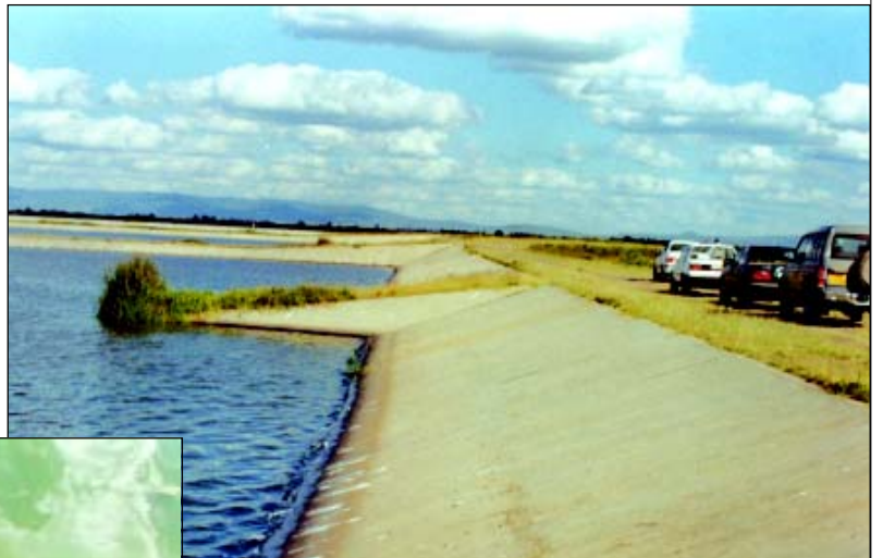
Plate 15. A part of the large secondary waste water treatment ponds at Ruai. The water has a reduced BOD and lower coli form count than that in the primary pond.
