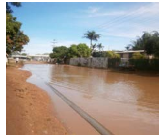
Poor drainage system resulting in overflow of water onto the road at the Rainbow residential area. Photo © Miria, G., 2012
