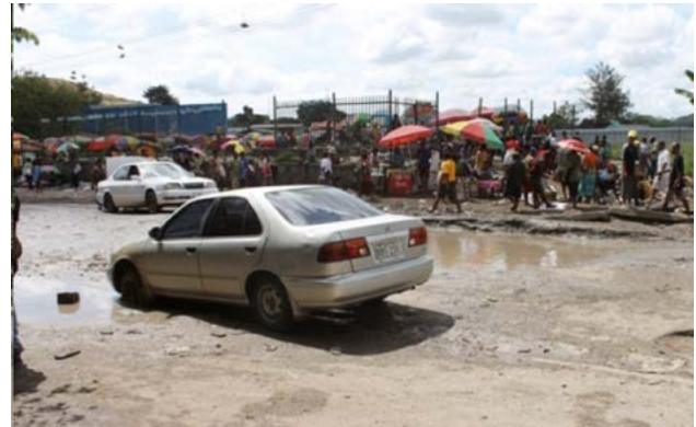
The impact of flooding on roads in the Gordons Area Photo © Goije, B., Kioma, T., Bobora, N., Bomai, A. and Kamaso, D. (2012)
