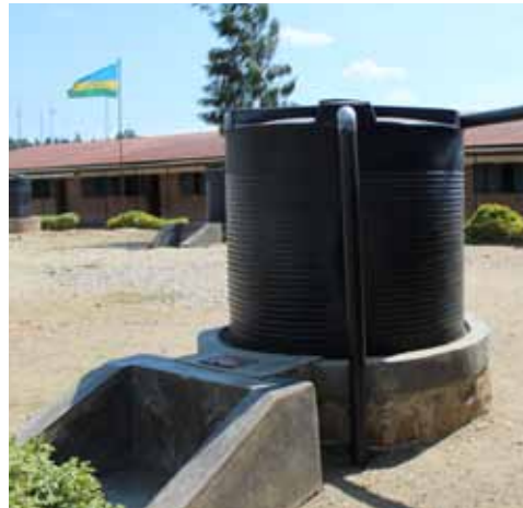
Rain water harvesting system installed in Kibuye high school © Arianna Francioni
