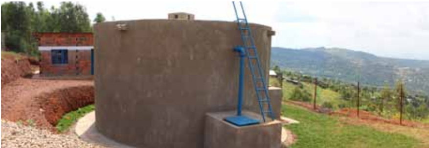
Water distribution reservoir in Gatenga sector © Arianna Francioni
