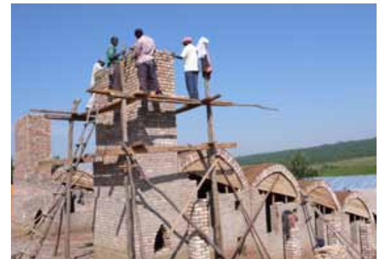
Local builders working at a tile furnace
