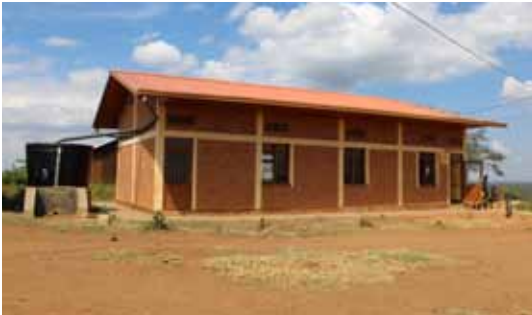
An energy kiosk with rainwater harvesting system
