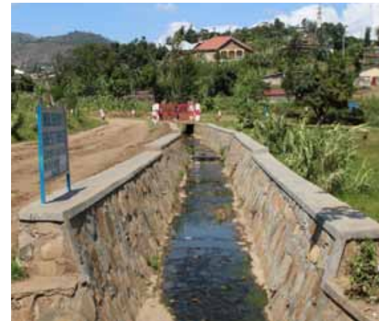
Bridge and drainage channel built in Karongi © Arianna Francioni
