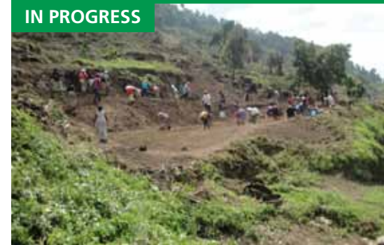
Rehabilitation process on Rubavu Hillside © UN-Habitat Office in Rwanda
