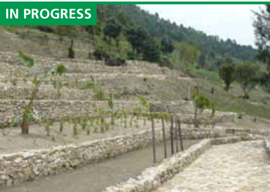
Rehabilitation process on Rubavu Hillside © UN-Habitat Office in Rwanda
