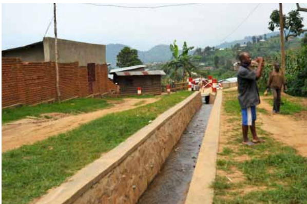
New drainage channel built in Karongi © Arianna Francioni
