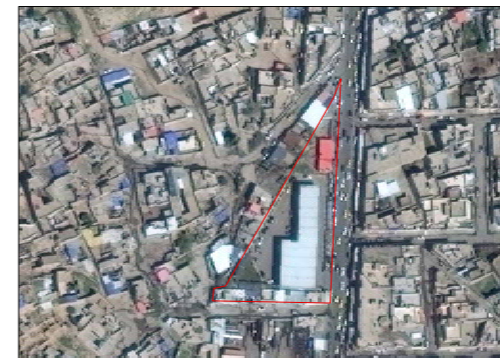
2 - Al Kuwer garage on Al Kuwer road East Mosul to Guer, Hatra, Gayar
