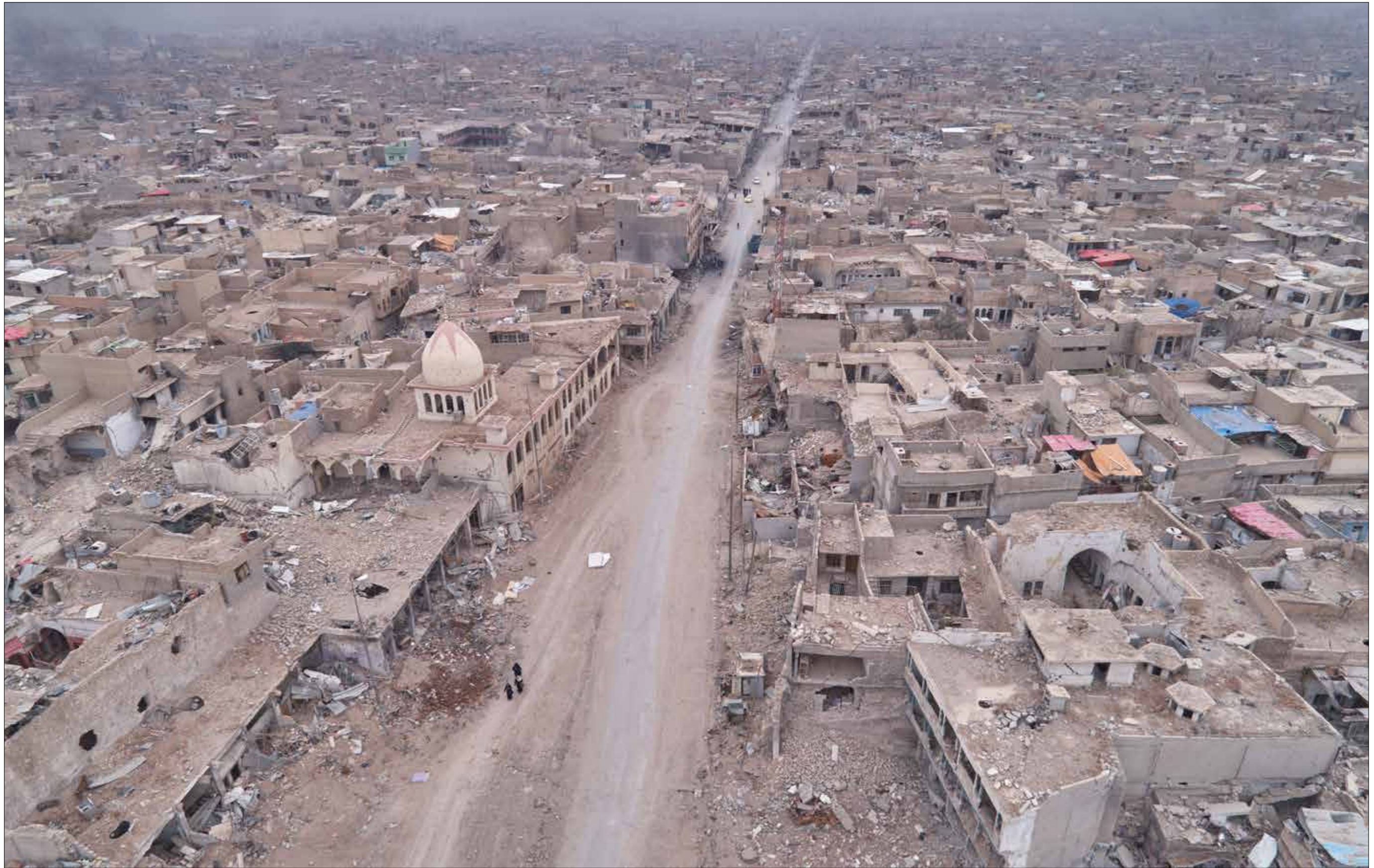
FIGURE 135. Even before the conflict, the Old City, with its dense urban fabric, lacked the space to introduce new facilities (UNESCO/ Iconem, drone imagery 2018)
