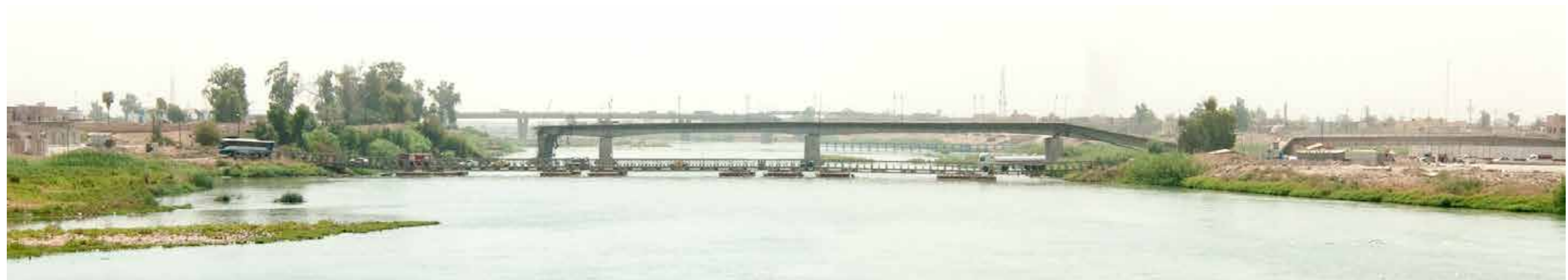
FIGURE 42. The temporary Al Huria Bridge (Victory Bridge) over the Tigris River (UN-Habitat/ Jan Willem Petersen, 2018)
