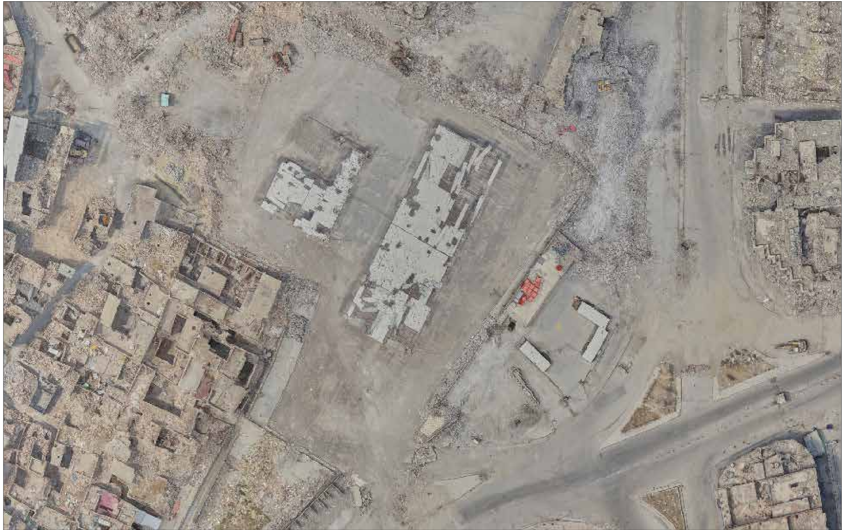
FIGURE 141. Damage to the right Bab Al-Tob Terminal in the Old City (Satellite imagery 2018/ UN-Habitat)
