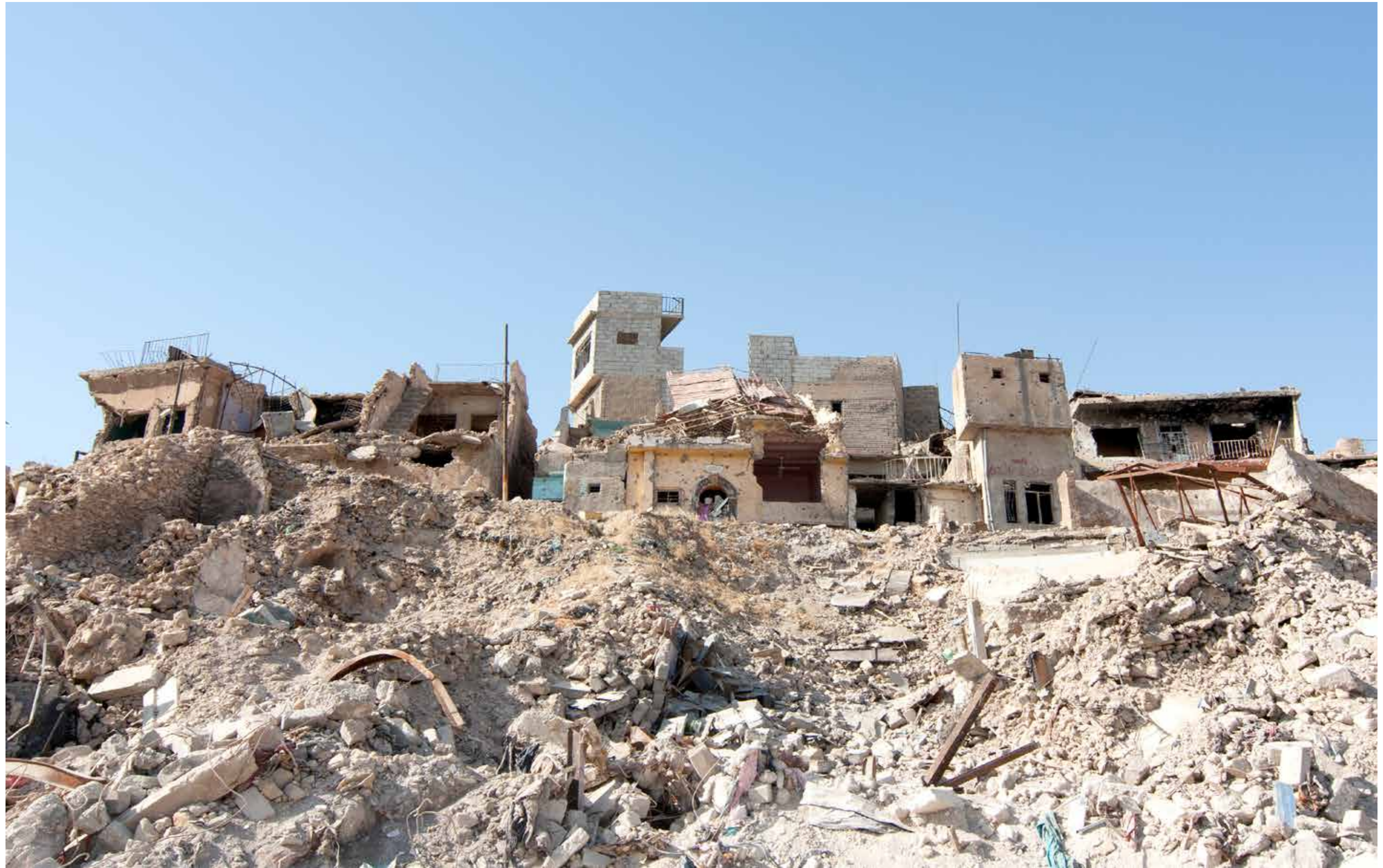
FIGURE 109. Extensive destruction of the Al Maidan area. For the Old City, debris and ERW clearance are intrinsically linked (UN-Habitat, Jan Willem Petersen, August 2018)
