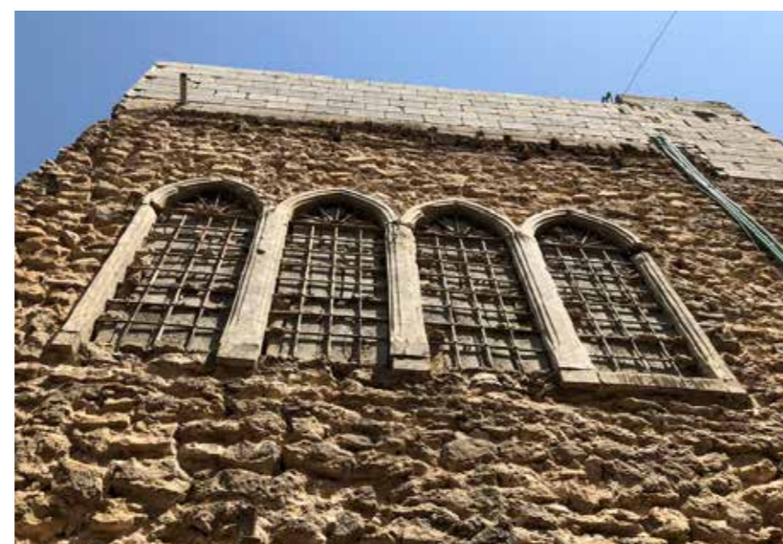
FIGURE 127. Ongoing reconstruction in the Old City Example of the result of residents not having access to traditional building material (UN-Habitat, Ivan Thung, August 2018).
