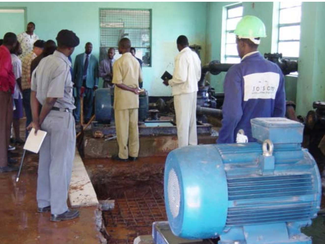
Inspection of the booster pumps. Photo © UN-Habitat
