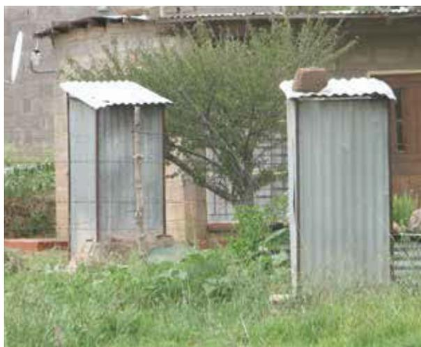
**FIGURE 62** VIP toilet showing vault at the rear. Most ventilation pipes are white instead of the recommended black so that they would be hot.
