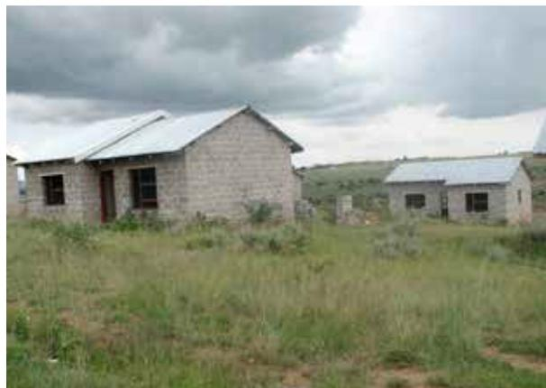
FIGURE 83 Complete experimental Hydraform block dwelling built by MLGCPA
