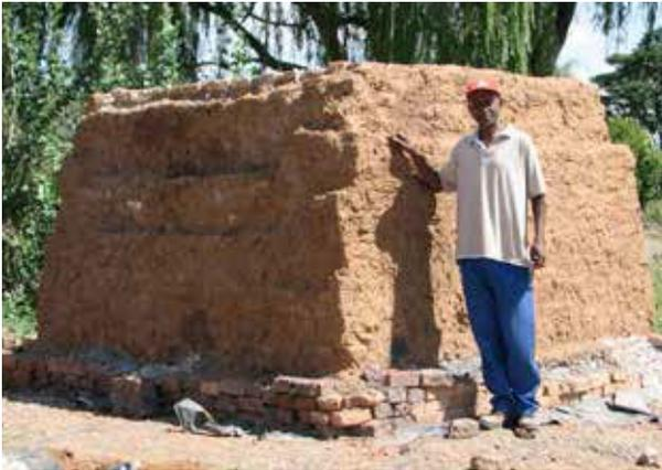
FIGURE 80 Local burnt brick used in *malaene*
