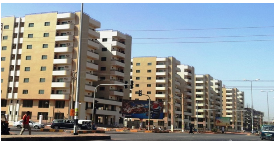
Example of newly-built multi-family, multi-story housing in Khartoum. Photo© UN-Habitat
