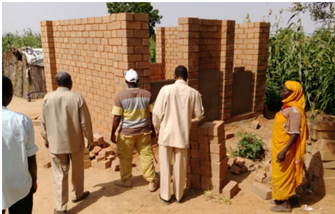
Construction of Self Help Housing in Anjemi village, West Darfur State. Photo© UN-Habitat
