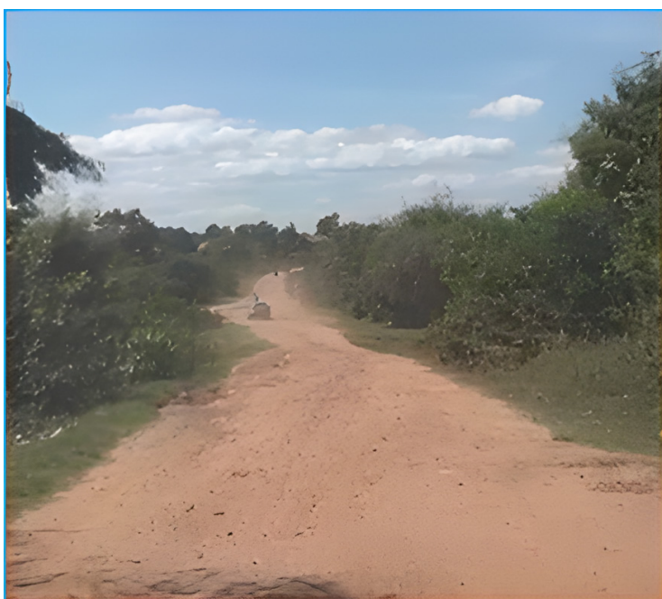
Main road access to Kaengsun village
