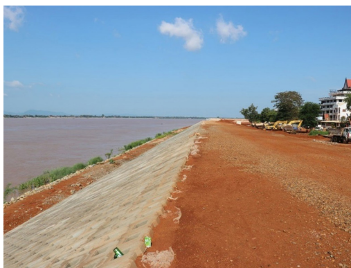
Construction of Mekong levee in 2020 [vientianetime, 2020]
