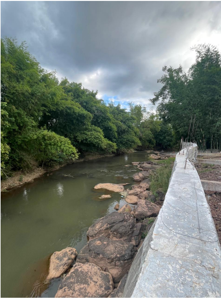
Local initiative to protect flood from the natural creek in Nahaek village
