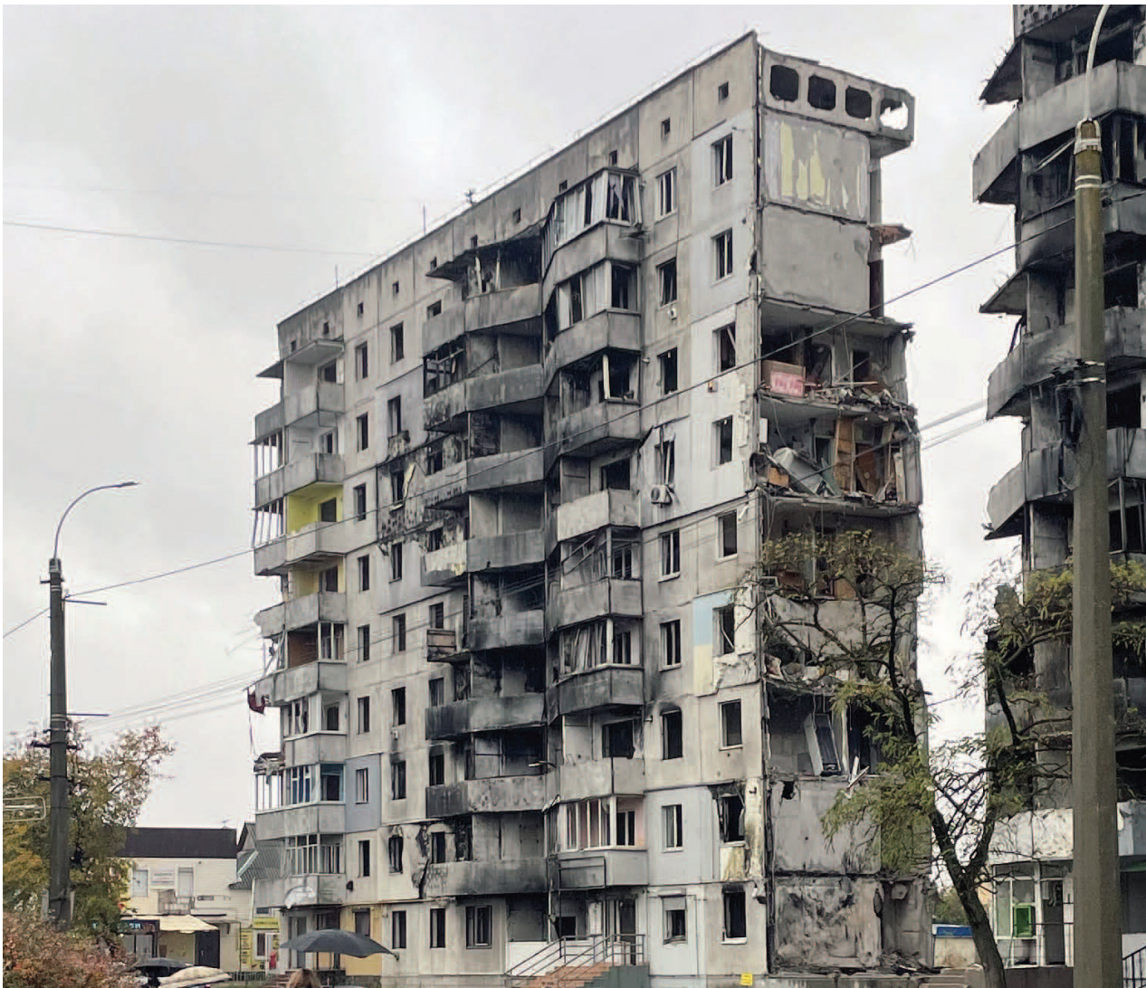
War damaged apartment block in Borodianka © UN-Habitat Ukraine
