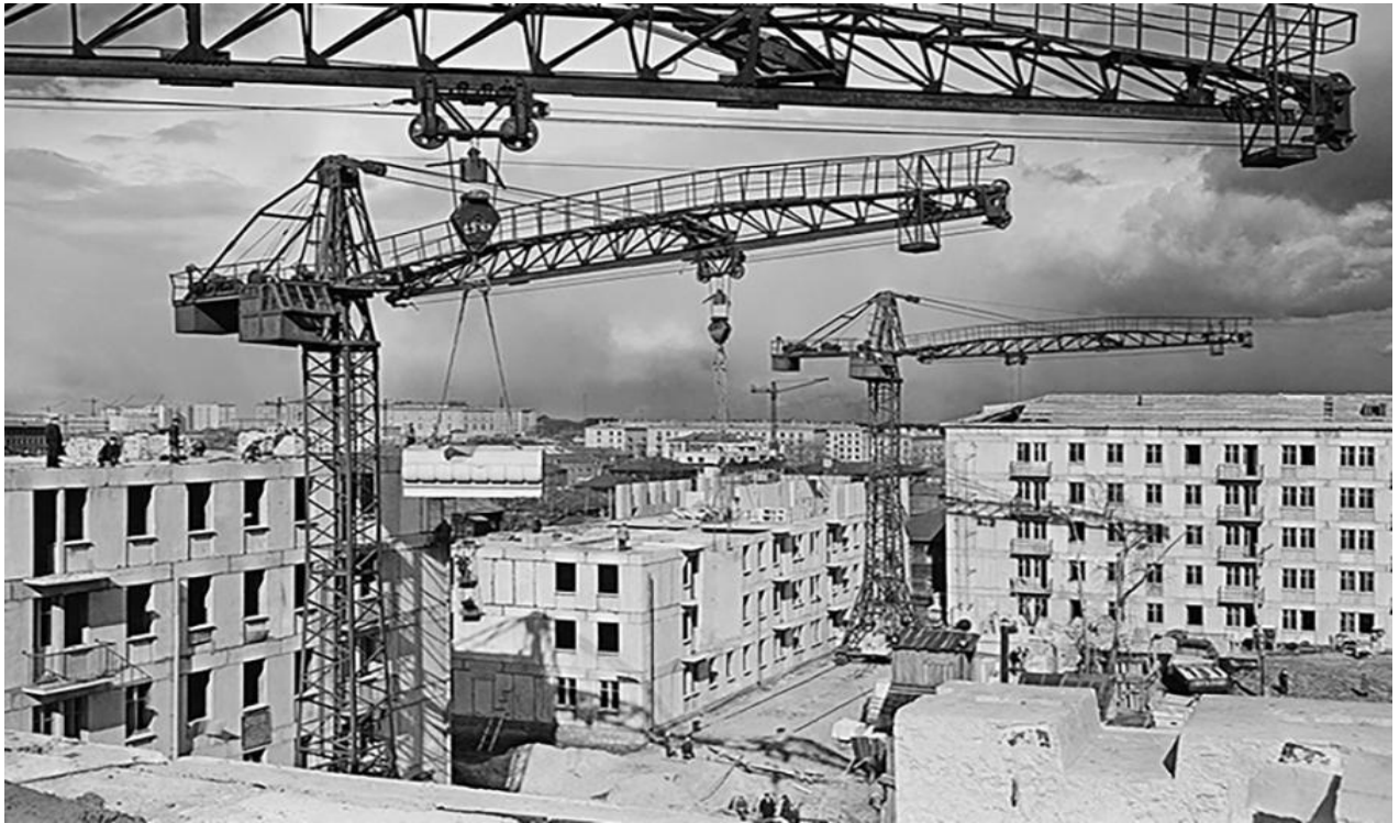
Figure 3: Khrushchyovkas - buildings with simple, repetitive designs, often grouped into large complexes. Photo: Kievinform.
