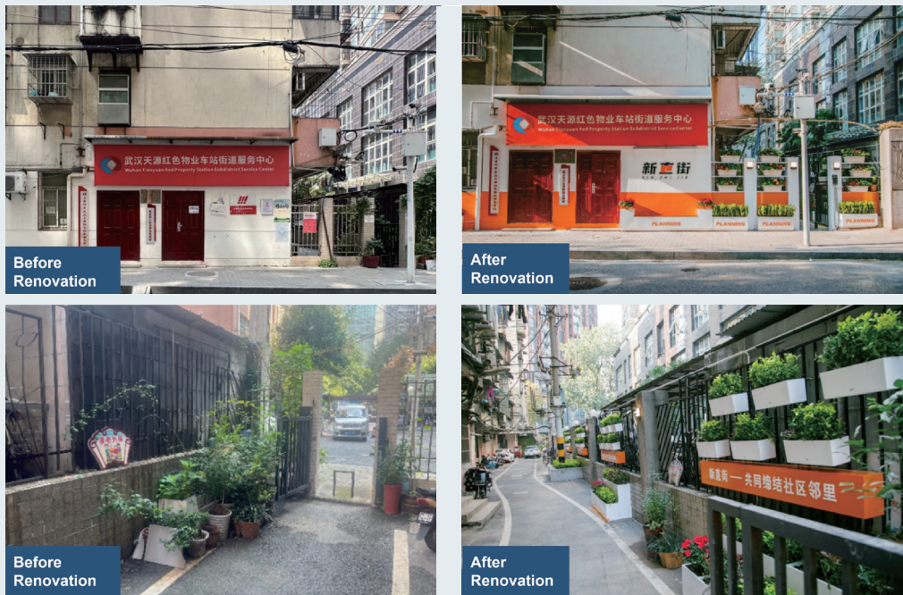
Figure 3.14 Comparison Before and After Renovation
