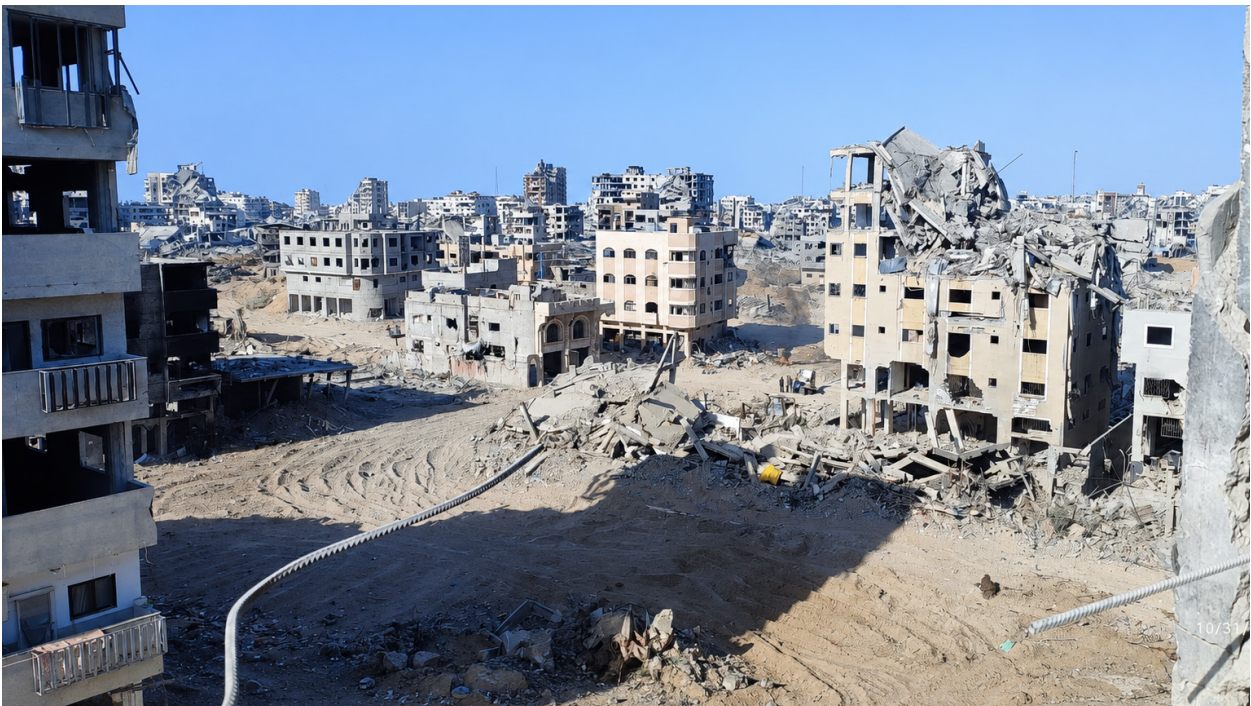
Figure 2.7: Extensive damage to residential buildings in Tel Al Hawa
