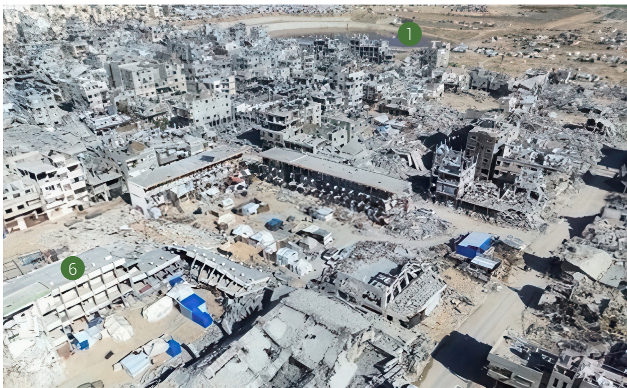
Figure 2.7: Emerging makeshift sites in relation to damaged public facilities
