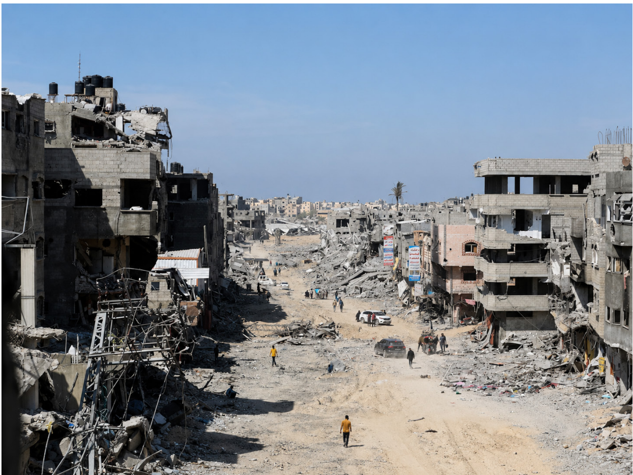
Figure 2.22: Damage to roads and built environment in Al Amal Neighbourhood, Khan Younis.
