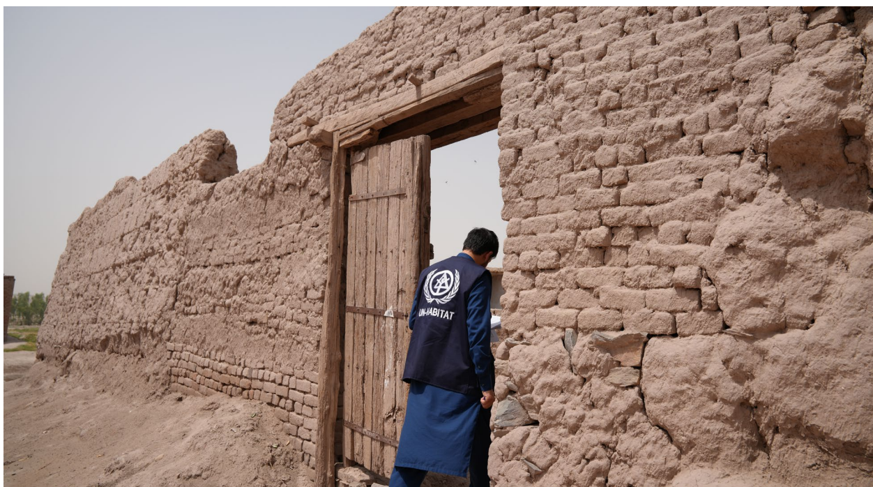
UN-Habitat engineer assessing shelters in Nangarhar, June 2025. ©UN-Habitat
