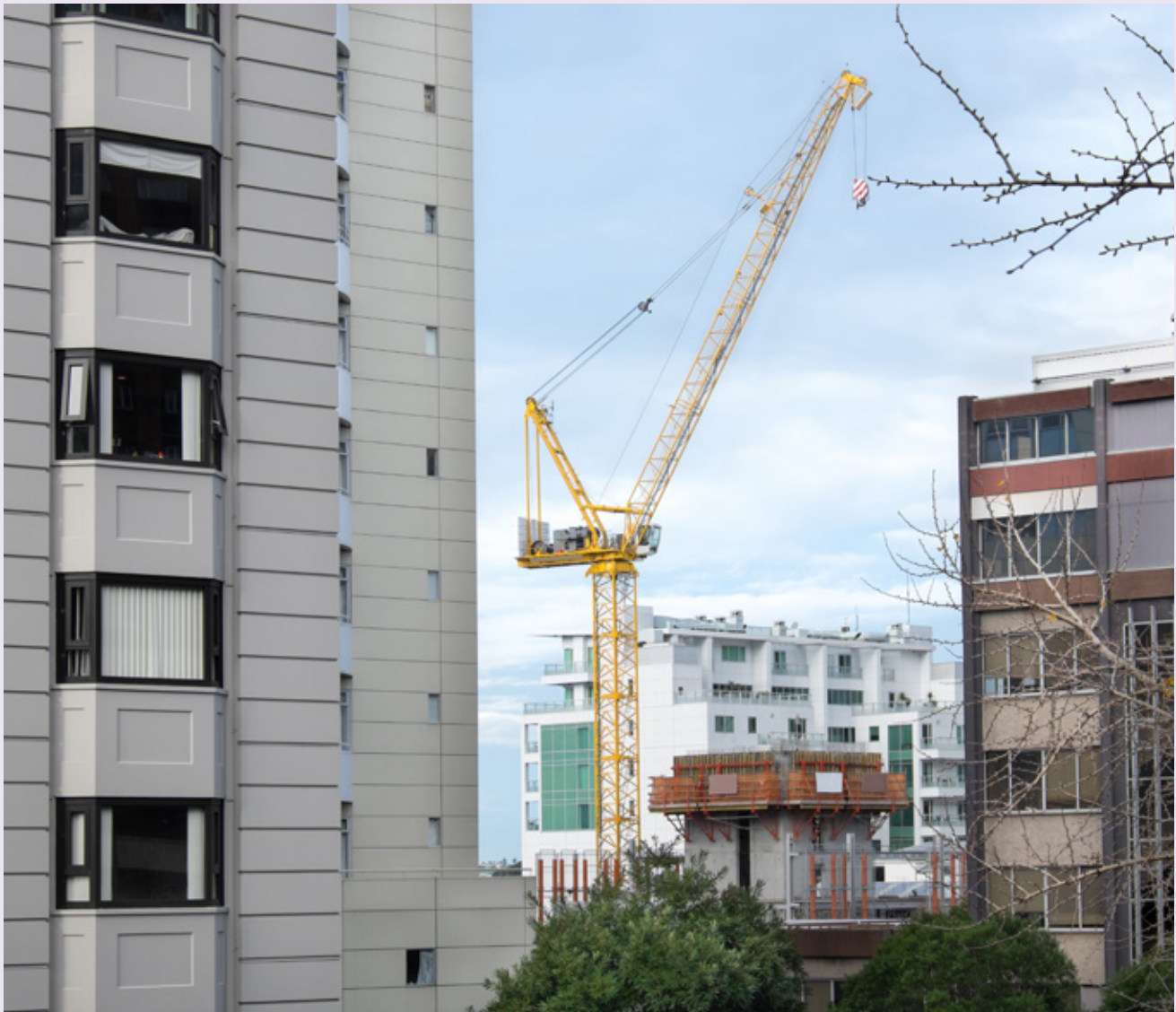
Apartment construction in Auckland's central business district, New Zealand. Photo: corners74/Shutterstock
