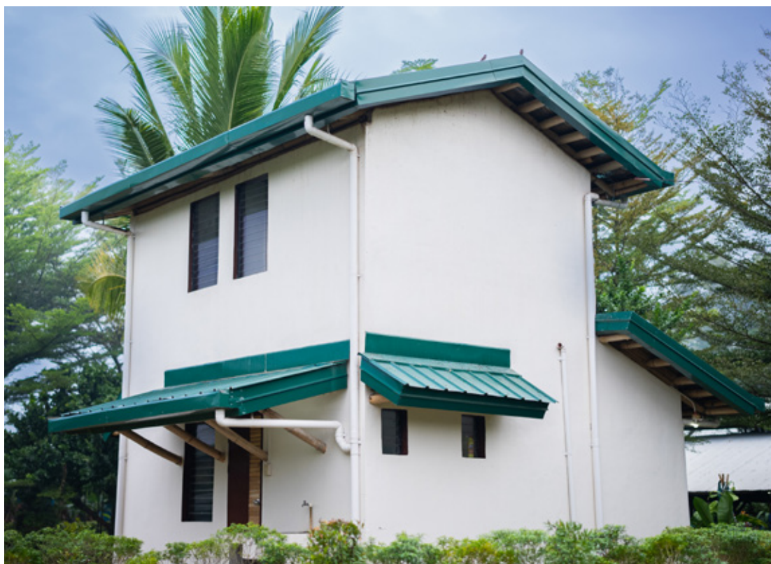
A home built using composite bamboo shear walls, combining locally available bamboo with low-carbon, hazard-resilient construction. Photo: Arup
