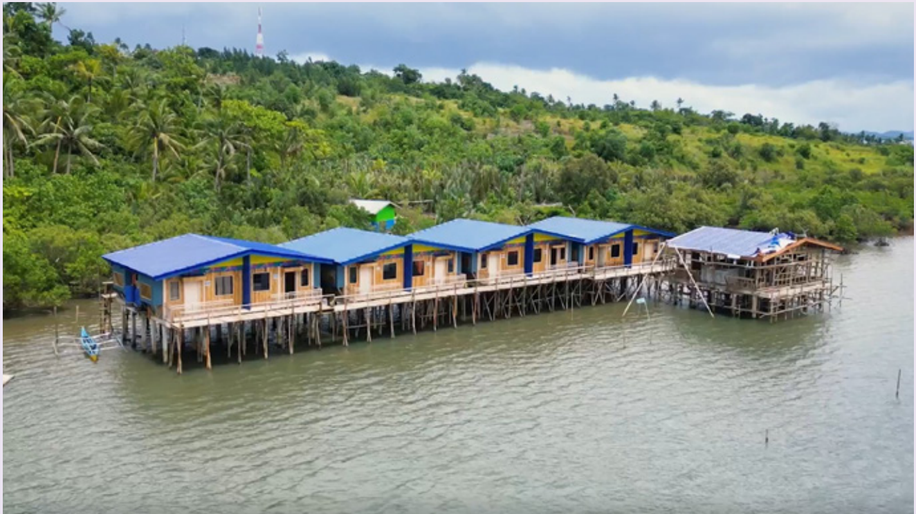
Climate-resilient stilt homes in the Huy-anan nan Bajau ecovillage in Surigao City, Philippines, designed with the Sama Bajau community to support culturally appropriate coastal living. Photo: UN-Habitat.
