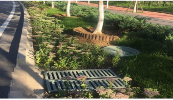
Riverside Avenue Pervious Concrete
