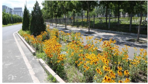
East Road High Bearing Permeable Paving
