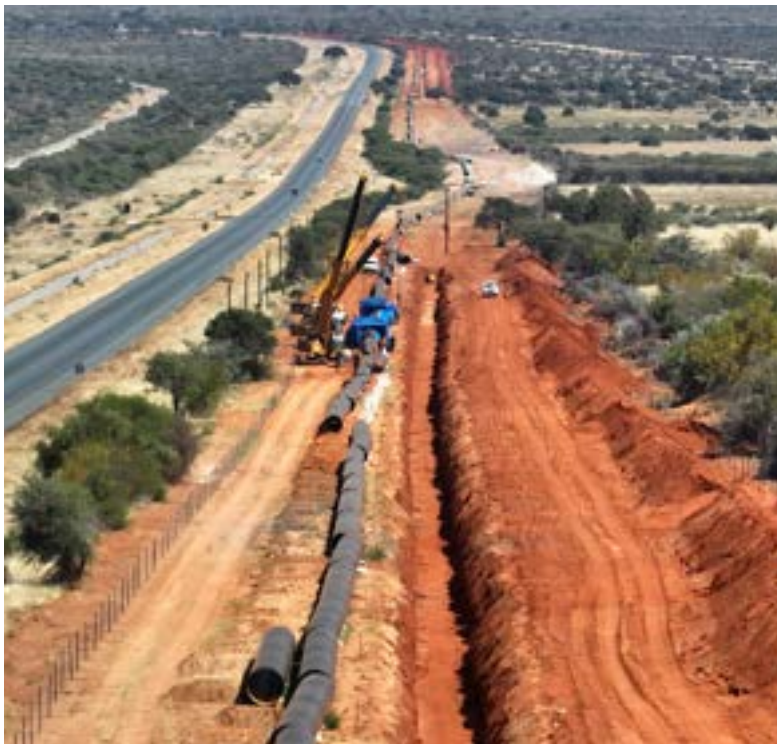
Water pipeline construction on the A1 highway, Botswana. © Shutterstock/Bashi Kikia
