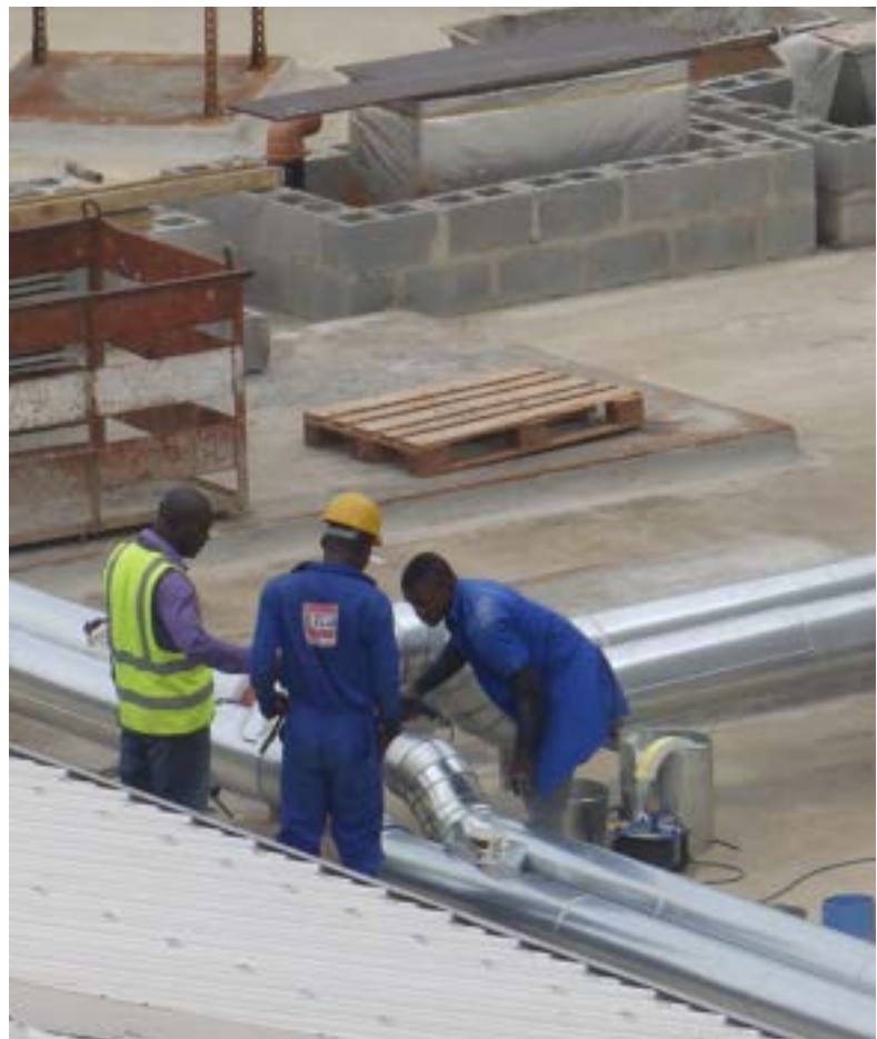
Installation of essential building systems in Lagos, Nigeria. © Shutterstock
