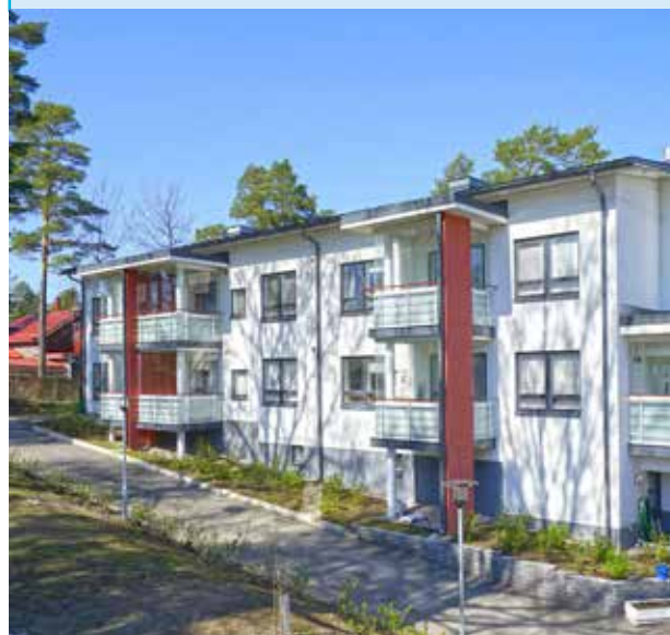
Väinölä supported social housing unit in Espoo, Finland. © Y-Foundation (Y-Säätiö)
