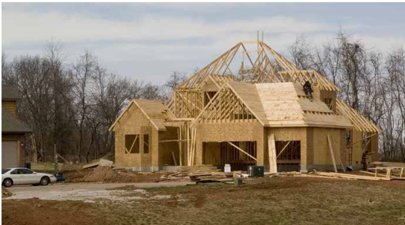
A new home under construction © Shutterstock
